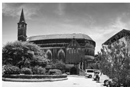
The Anglican Christ Church, a landmark monument in Zanzibar and a prominent example of early Christian architecture in East Africa (1873-1883). mixing perpendicular gothic and Arabic details As most buildings in Stone Town, it is made mostly of coral stone.
